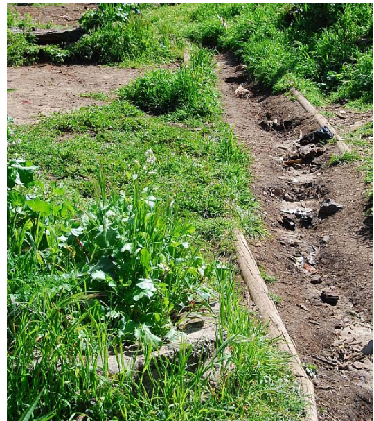
Trail erosion caused by overuse creating a depression followed by water channeling.
